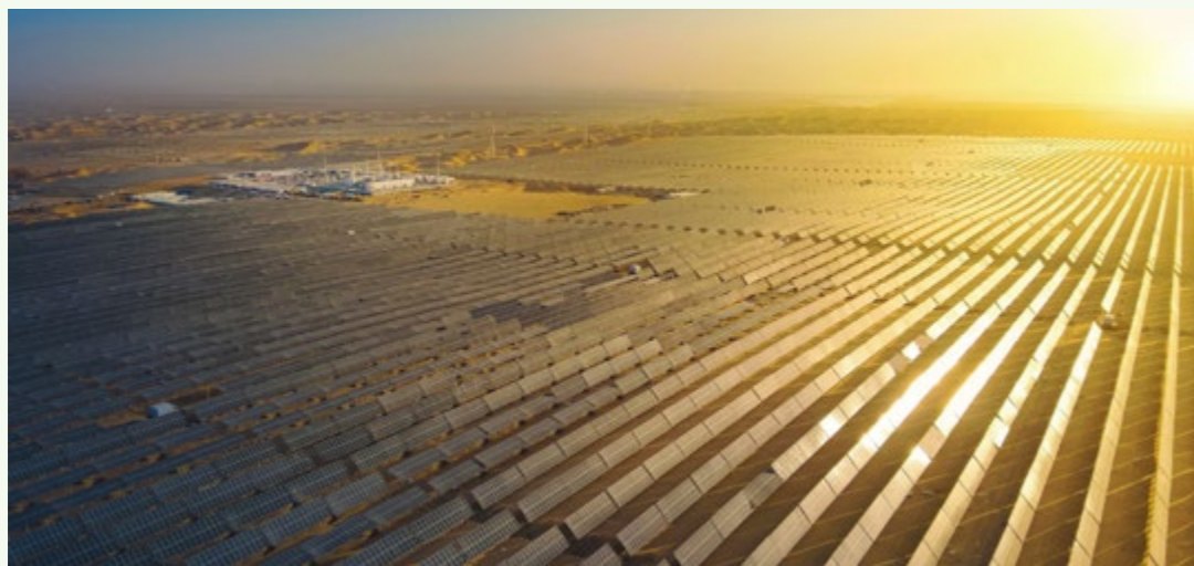
▲ Ningxia Branch supports the Zhongwei photovoltaic project. (Photo provided Ningxia Branch)
