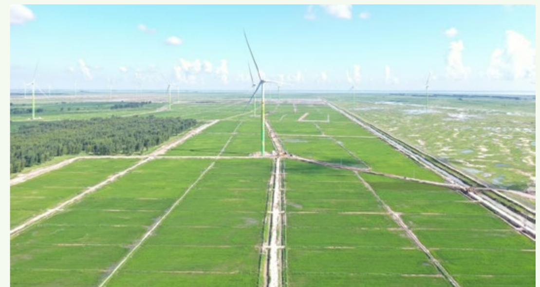
Beijing Branch supports the saline-alkali land improvement projects. (Photo provided by Beijing Branch)
